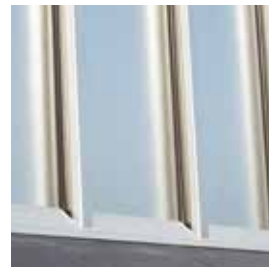
Rubber infill strips to prevent the lodging of dirt and debris.
