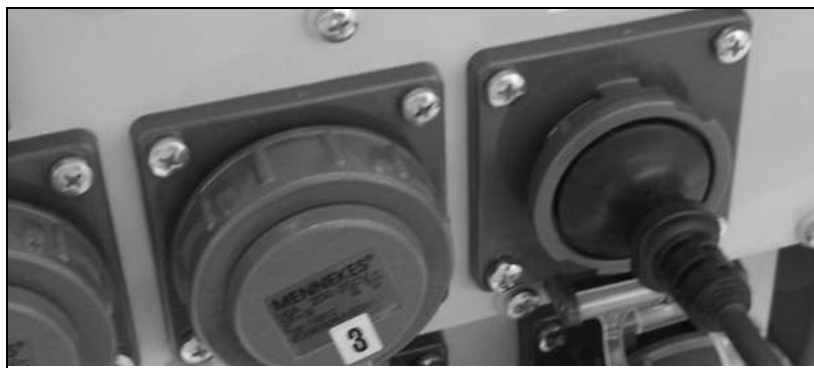
Fig. 4-4: Connecting up consumers/appliances
