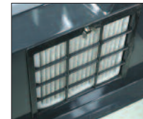
Recirculation air filter
